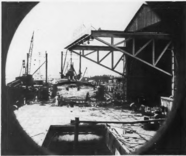
THROUGH PORTHOLE, conversion on deck of former Navy LST makes a busy picture. Work is expensive, takes several months for each ship.
